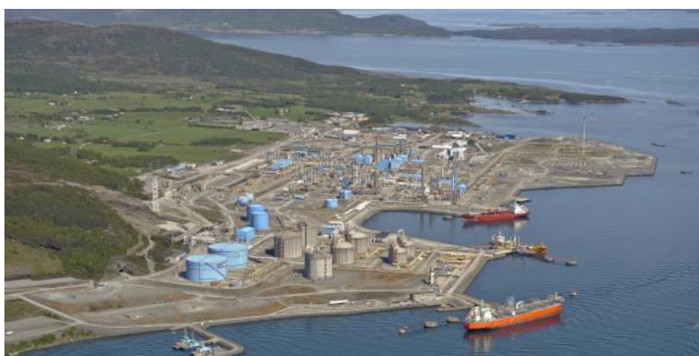
Figure 27: Picture of the gas and condensate processing plant at Kårstø (Source: Norwegian Petroleum, Photo: Øyvind Hagen-Gassco)
